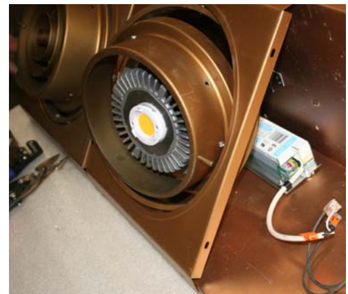
P56-LB LED Par Lamp Retrofit installed in an existing triangle corner unit. Remote driver features magnetic feet for "no screws needed" mounting.
